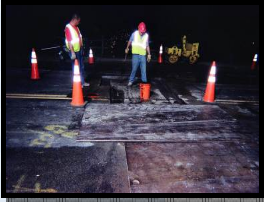
Utility Construction Work on State Right-of-Ways
